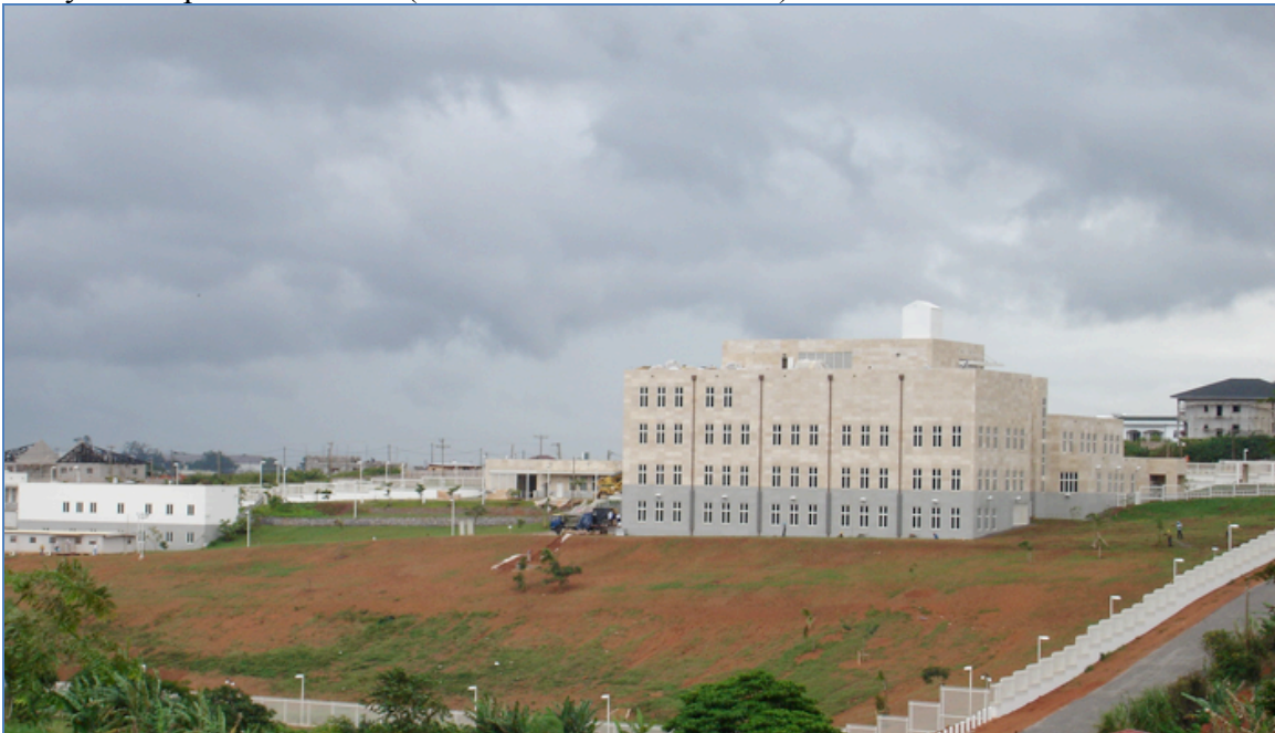
FIGURE 2. The new normal. Construction on the new U.S. embassy in Yaoundé, Cameroon, in a sparsely populated new diplomatic enclave. Note the large lot and setback space; perimeter walls with flood lights; and fortress-like structure with narrow, likely bullet-proof windows (Caddell Construction ND).
